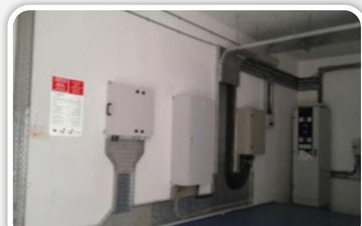
DMS Panel Installation and termination at Sigma 1
