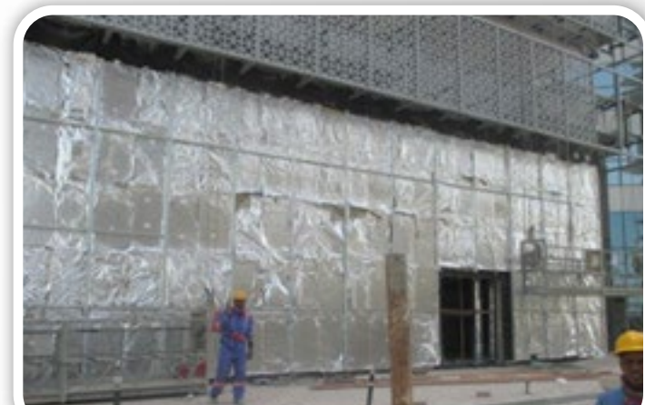
Mashrabia panel & ACP installation podium levels
