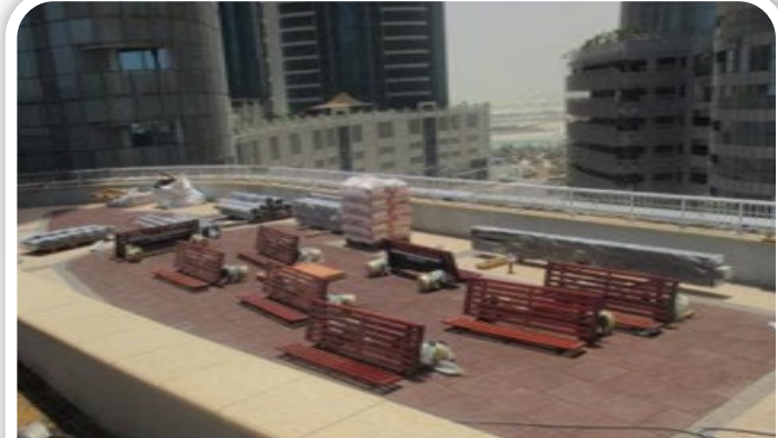
Swimming pool area wooden benches installation
