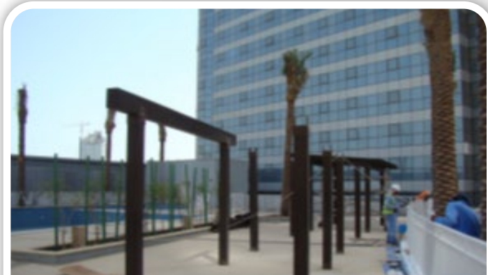
Podium Level swimming pool handrail painting
