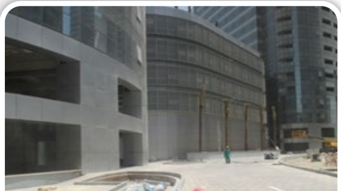
Road side ground level paving works
