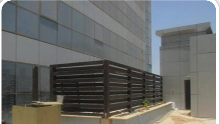
Swimming pool timber trellis installation
